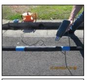
The end masking tape can be removed with Stanley knife or similar.
